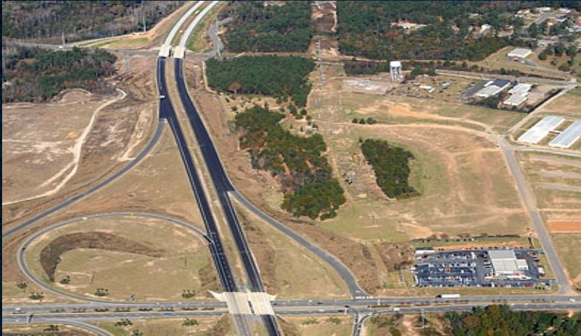
Aerial view of I-520 north from US 1 to Powerhouse Road (December 2009)
