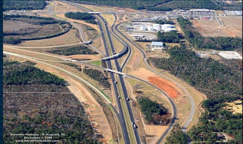
Aerial view of US 25 and completed bridges on I-20 (December 2009)
